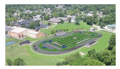
**Pictured:** Rendering shows the proposed Brown County High School football field and track shifted out of the Greasy Creek floodway, with a raised turf field, post-tension track, new home grandstand and relocated visitor seating. Concessions and restrooms are moved closer to fans for easier access. **Rendering provided by Tarkett Sports Design**
