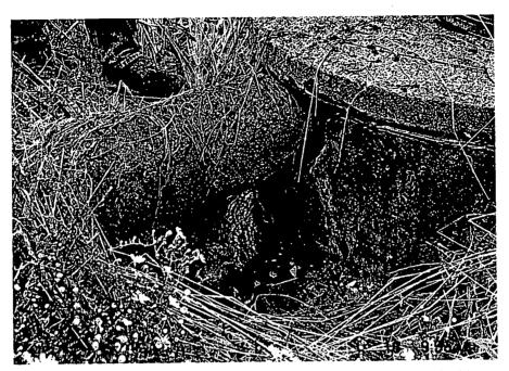
Figure A4: A view of one of the mobile home park's septic tanks, looking southwest. Notice the dark wastewater being discharged from the tank. The trailer court is located to the left, uphill of this scene.
