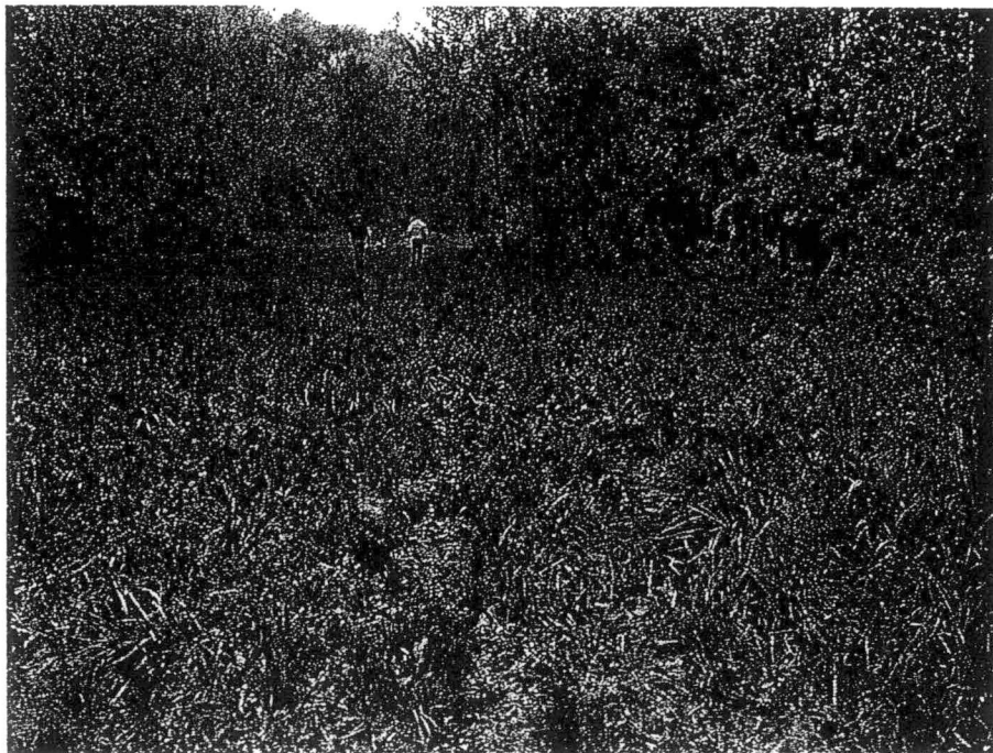
Figure A6: A view of the trailer court's leach field, located west of the septic tank shown in Figure A4. Again, dark wastewater and abnormal plant growth are present.
